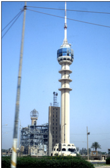
Fig. 15. Telecommunications(?) building, destroyed by pinpoint bombing (© J. Russell)
